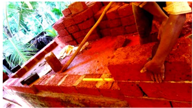
Figure 5: Masonary with Laterite stone and Surkhi Mortar
