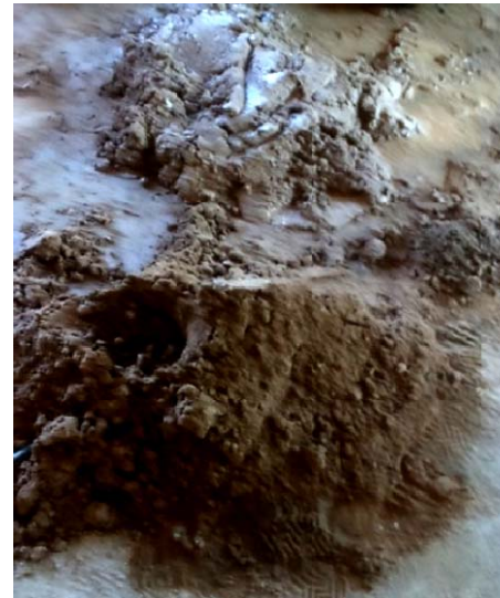
Figure 9: Mixing of Surkhi Mortar
