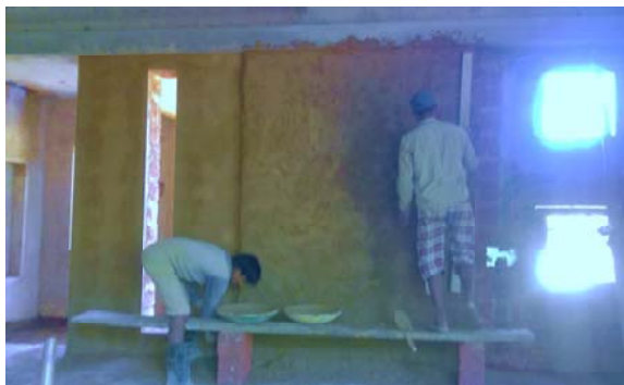
Figure 8: Internal wall plastering with Surkhi Mortar
