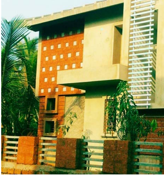
Figure 14: Façade look before painting
