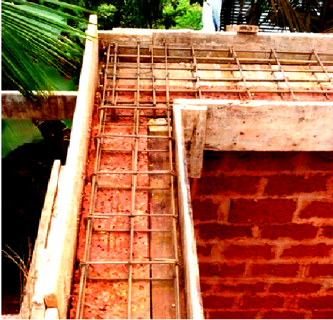
Figure 7: Special RCC Pad Beams along the Masonary walls
